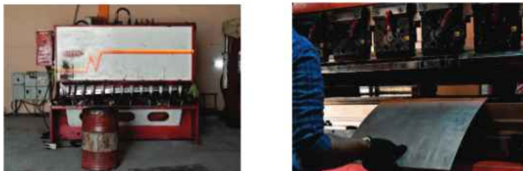
FIGURE1: Cutting & rolling of CRC Steel sheets
