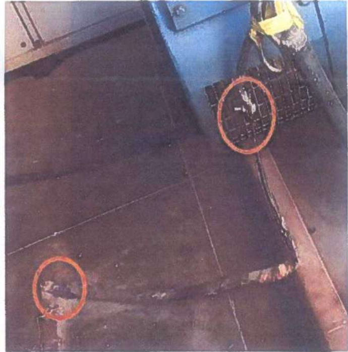
Earth pit NOT traceable, interconnections with Bolts not allowed, should be braised
